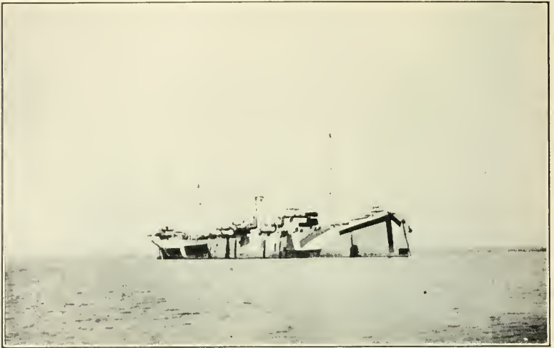
Photo from Bureau of Construction and Repair, U. S. N.
